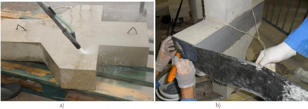
Figure 2: Details of bonding system of: a) Sandblasting of corbels and b) Application of carbon fiber on concrete surface by wrapping.
