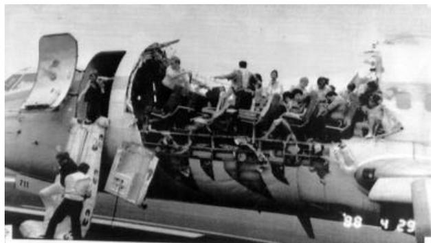
Figure 1. Fatigue crack growth in an aircraft structure.
