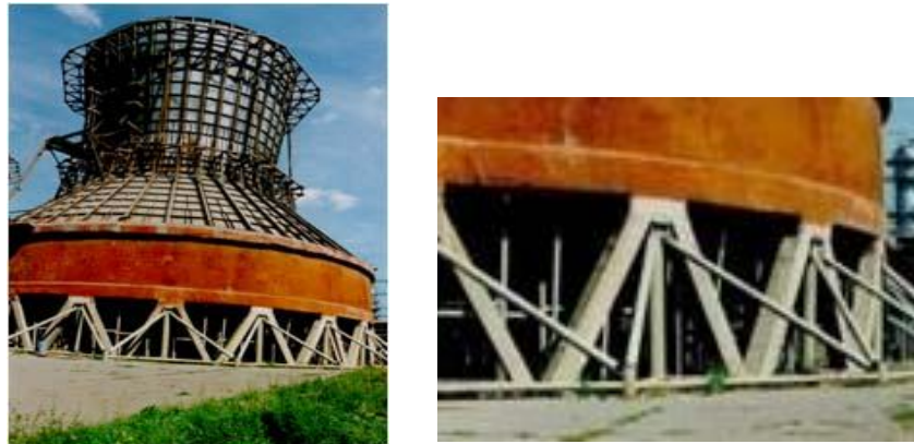
Fig. 4. Basic system for cooler SK-1200 strengthening
