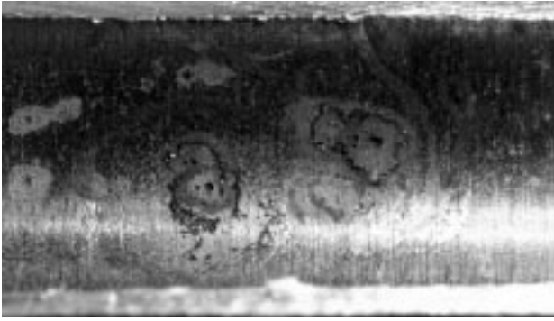
Figure 6: Pitting at the internal surface of the tubes
