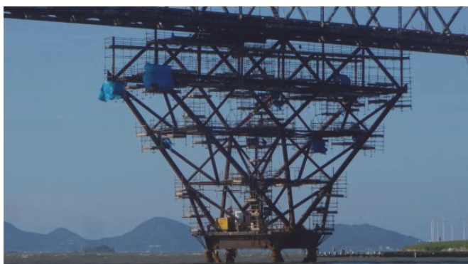
Figure 22: Auxiliary structure tower assembly.
