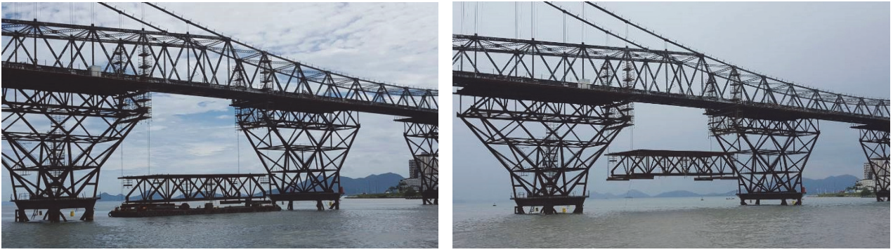
Figure 23: Transportation and hoisting of an auxiliary structure truss part.
