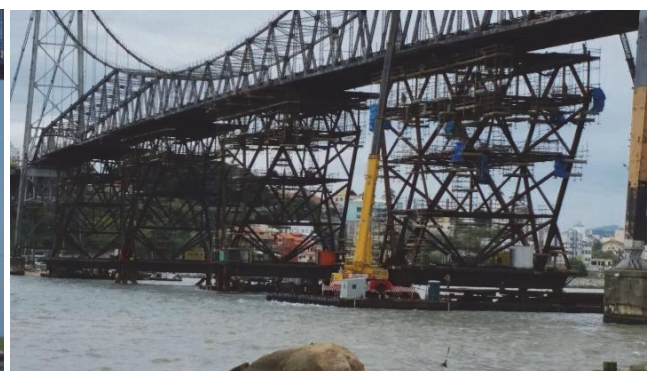
Figure 22: Auxiliary structure tower assembly.
