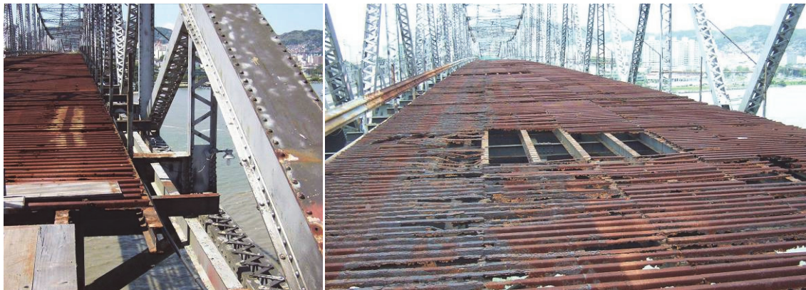
Figure 9: The high corrosion state of the steel deck.
