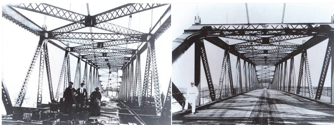
Figure 7: Deck photos (a) Support metallic elements assembly (b) Complete main span deck [19].
