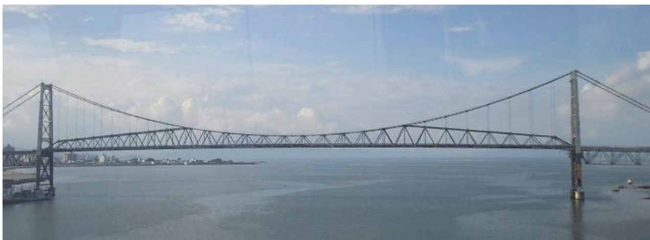
Figure 1: Main span of the Hercilio Luz Bridge (339.5 meters long).
