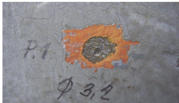
Figure 11: Hardness test in main structural elements.
