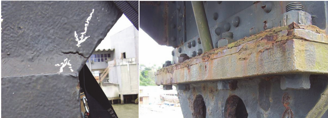
Figure 8: Fissures and the high corrosion level at the pylon base.
