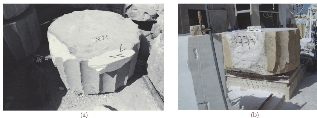
Figure 7: (a) Titanium bars are inserted from the upper side of the supplement used to fill the first mass loss after its fitting with the main volume of the drum. The second fracture is discernible on the left. (b) The supplement used to fill the second mass loss is joined to the main volume with horizontal internal titanium bars.
