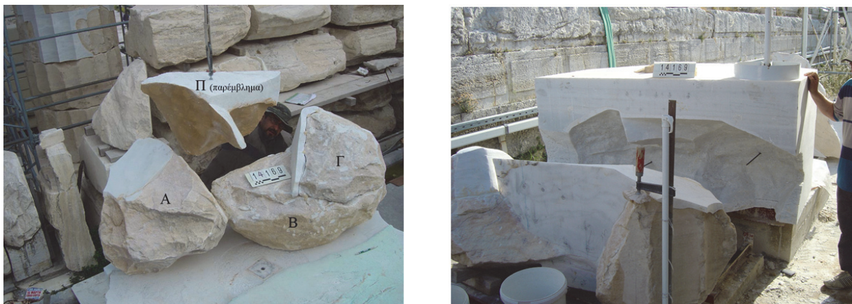
Figure 1: Joining together the ancient fragments A, B, Γ, with the new insert Π to keep them in the right position within the member's volume using cement mortar (left). The joining of this group and the main block of a new marble with "montage" reinforcement bars is presented in the right photo. In the foreground view the opposite fractured surface and the points, where reinforcing bars will be inserted during the next step of intervention, are presented. (Author's note: All pictures in this paper are from the archive of YSMA).
