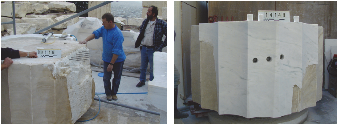
Figure 19: Inserting titanium bars on the upper side's area of the drum to join the supplement “D 1 F 1 ” to the ancient marble (on the left). After joining the supplement “D 1 F 1 ” to the main volume of the drum, the holes on its surface (in order to adjust the titanium plate anchor) sealed with the pieces of the extruded new marble (on the right).
