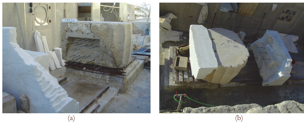
Figure 12: (a) Joining the first supplement. (b) Joining the second supplement. On the left the first –raw- supplement is already joined.
