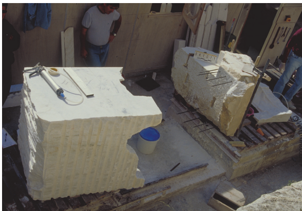
Figure 5: Joining the supplement A to the ancient volume (on the left). The supplement \Gamma with the proper reinforcement on it, is ready to be joined to the rest of the drum (on the right).
