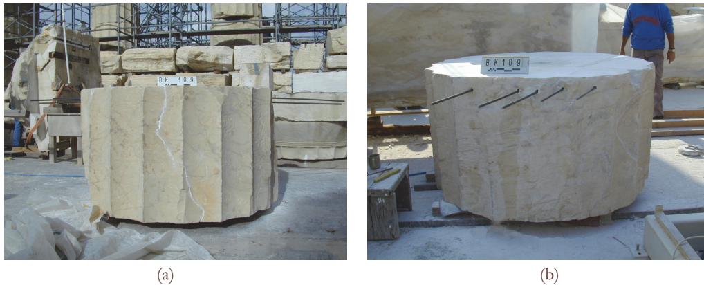
Figure 14: (a) View of the fracture plane. (b) Inserting the reinforcement on the lower side of the drum. In this picture the drum is upside down.
