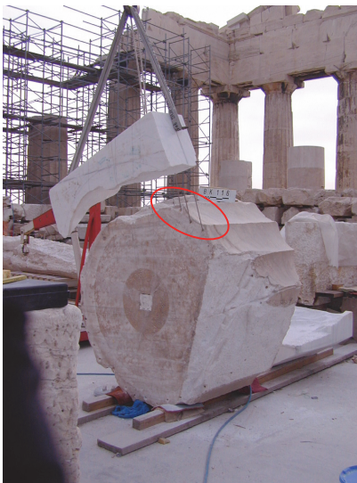
Figure 17: Adjusting a new marble (supplement “DF”) onto the upper side of the drum (left). Near by, the reinforcement required to restore the fragment “ \Delta FF_1 ” is presented (ellipse in the left figure). Drawing of the parts to be joined together and their geometry for the calculation of the stress field and consequently the reinforcement required (right) (Drawing: M. Mentzini, YSMA Archive).
