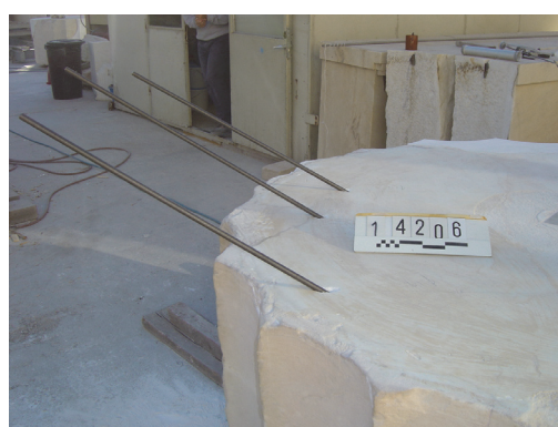
Figure 8: Titanium bars are inserted to repair the crack. In this picture the drum is upside down.
