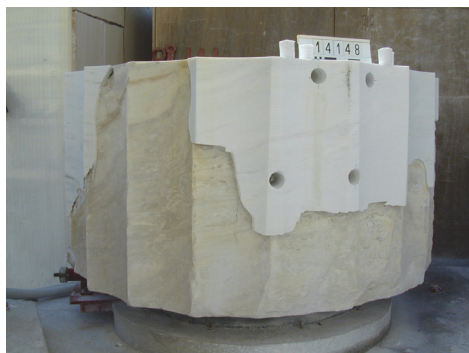
Figure 18: After joining the supplement “DF” to the main volume of the drum, the holes (in order to adjust the titanium plate anchor) on its surface sealed with the pieces of the extruded new marble (on the left). Repairing the crack “ df_2 ” (on the right).
