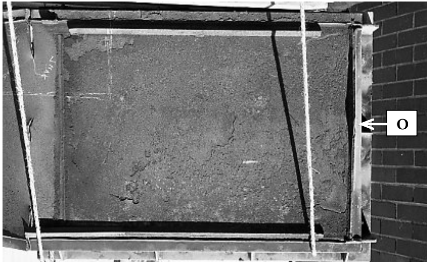
Figure 5: Fracture surface of the failed box section which led to collapse of the portal crane. The letter 'O' indicates the outer edge of the section, where the cracking started.
