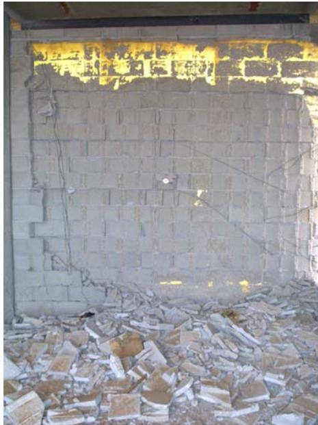
Figure 2. Complete destruction of masonry inside the West wall
